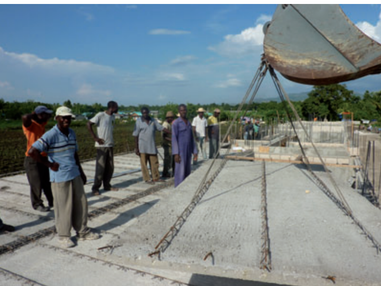
The precast flooring is transported to the site, where it is installed and concreted on site with simple equipment (images: Pro Haiti)
