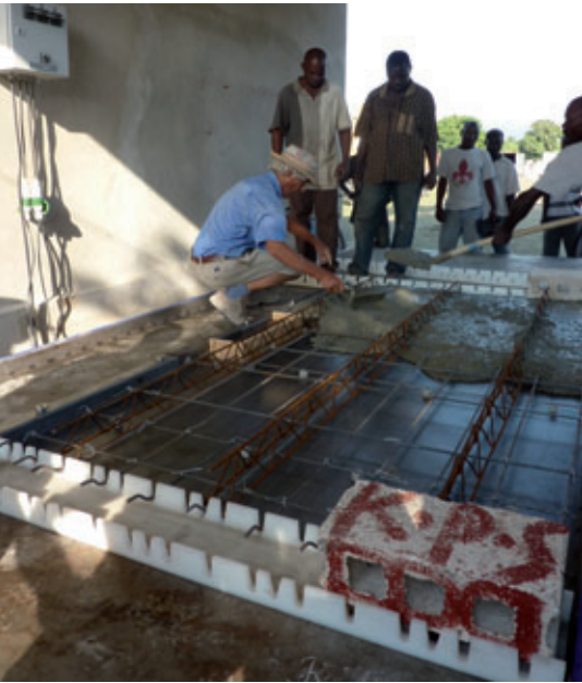
Precast flooring is produced on a stationary production table, provided by the German company Weckenmann (Images: Pro Haiti)
