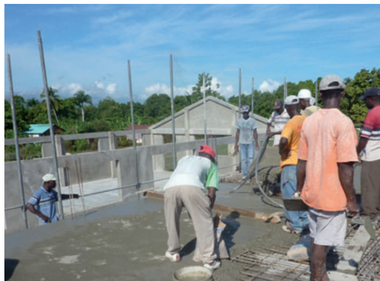
The precast flooring is transported to the site, where it is installed and concreted on site with simple equipment (images: Pro Haiti)
