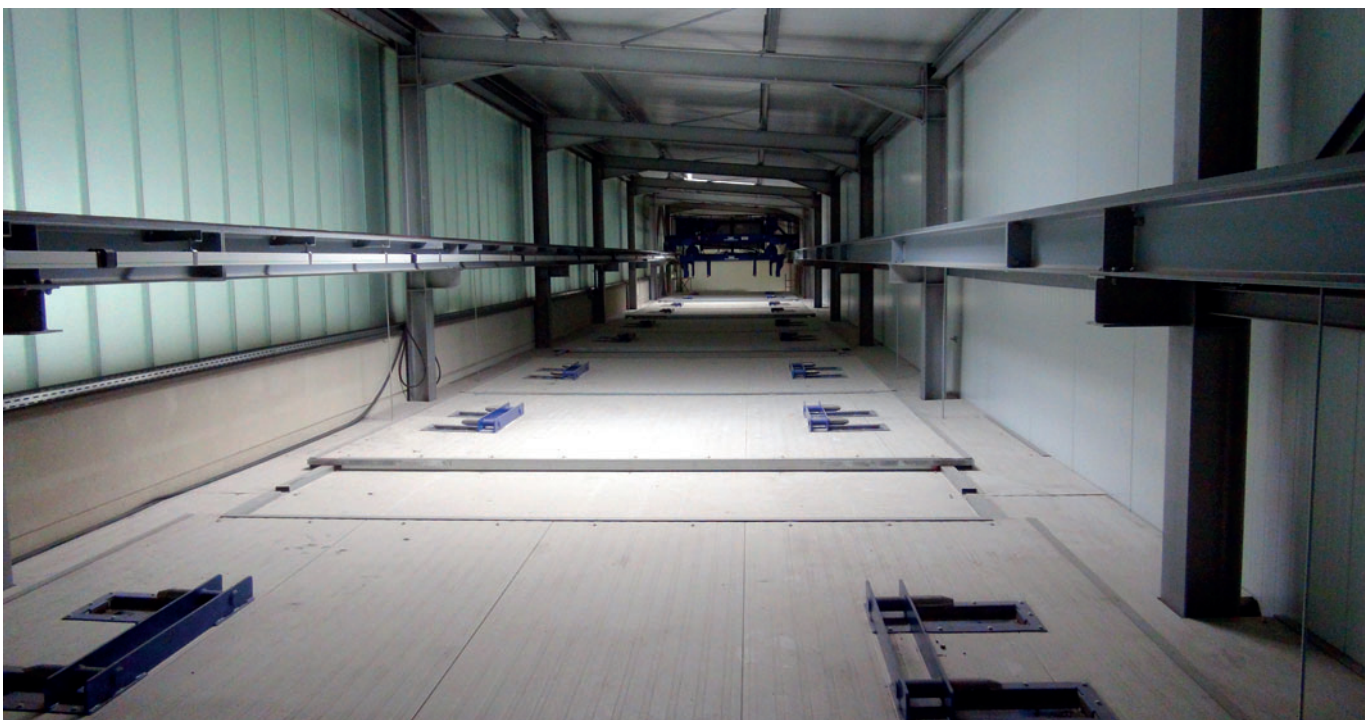
A look inside the new curing chamber at Rail.One in Coswig.
