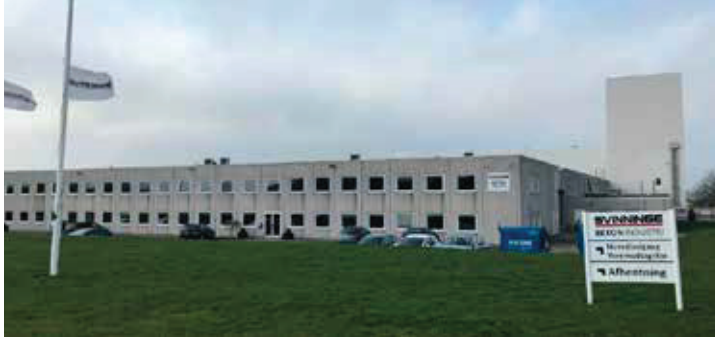
In 2018, the company Svinninge Beton Industri decided to integrate a new precasting plant in an existing building
