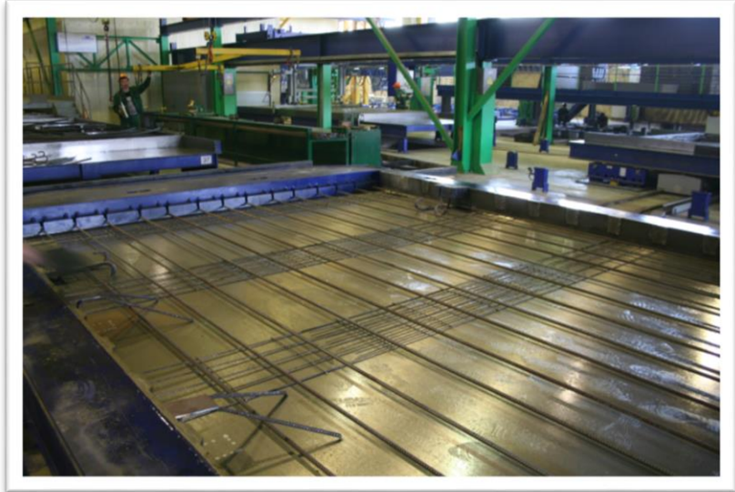
Prestressed with reinforcement bars
